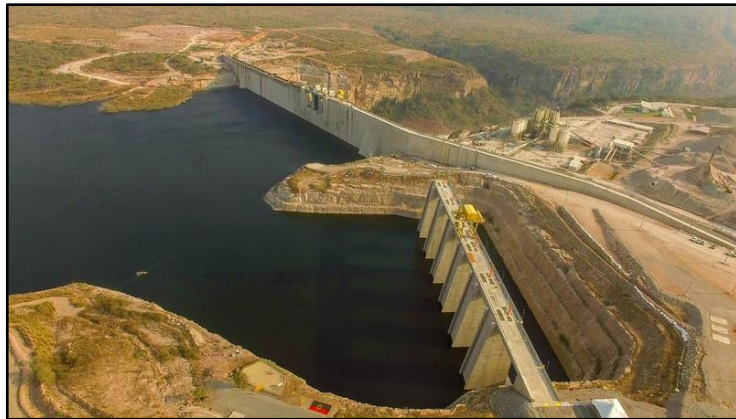
Figure 14: Angola's largest hydropower Lauca in operation Source: Lahmeyer International
