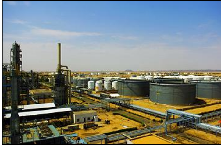
Figure 24: The Khartoum Refinery Co. Ltd. Installation is largest refinery in Sudan. Source: Time
